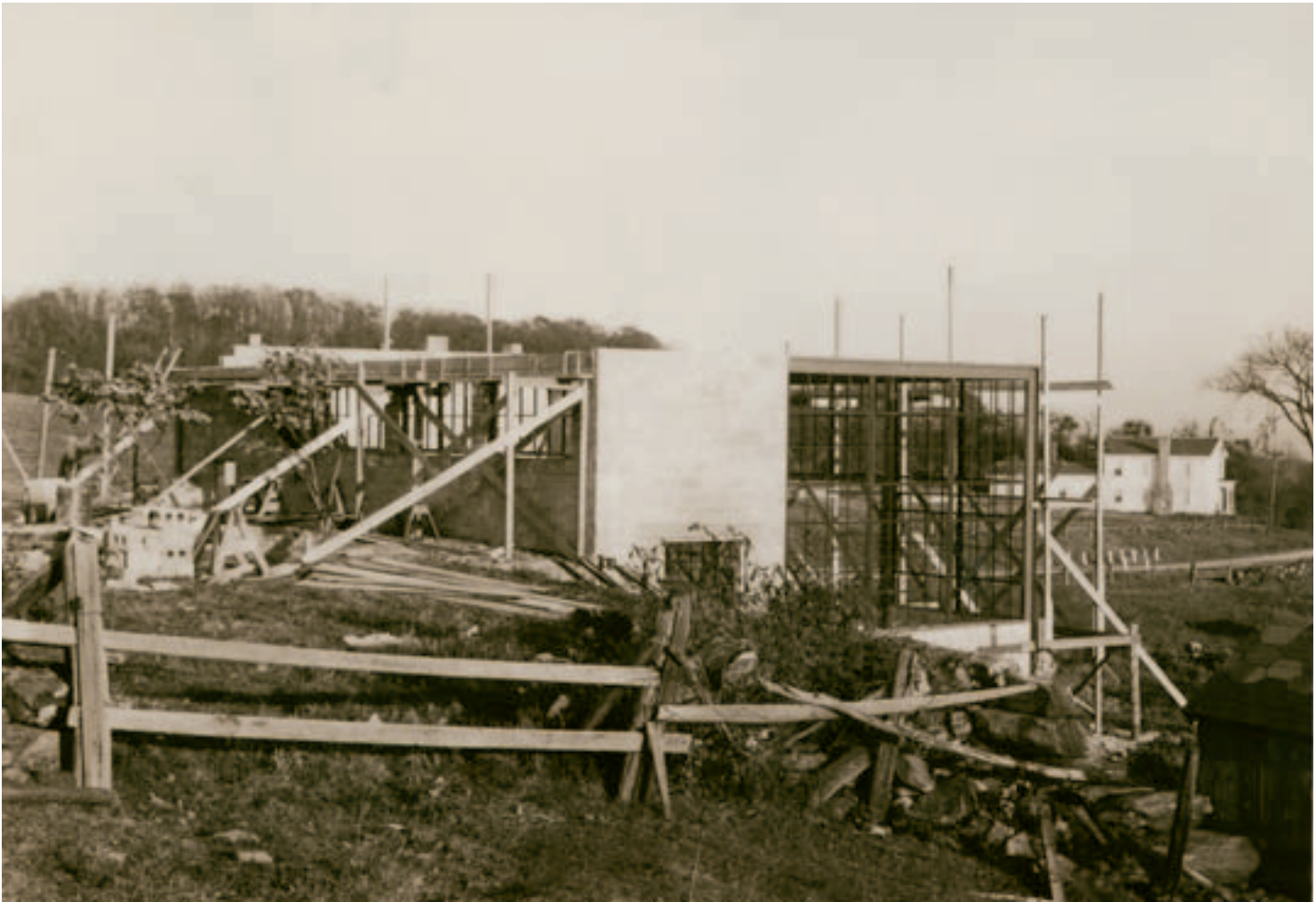
Construction of Calder's Roxbury studio, 1938
