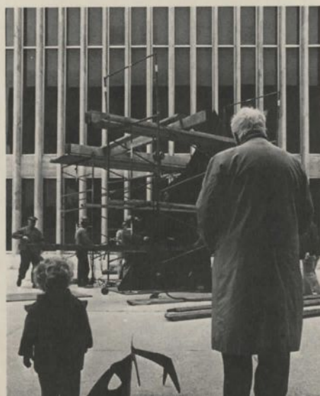
Alexander Calder and his grandson, Alexander Rower, survey the installation of Le Guichet at Lincoln Center, November 11, 1965. Calder's maquette for the sculpture is in the foreground. Photo: Bob Serating.
